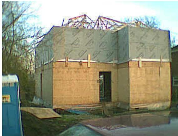
With 1st floor wall-panels completed, the "blockhouse" effect is even more obvious! Roof trusses for the hipped roof are going up quickly now using adjustable trestles to provide a working platform just below ceiling tie level.
