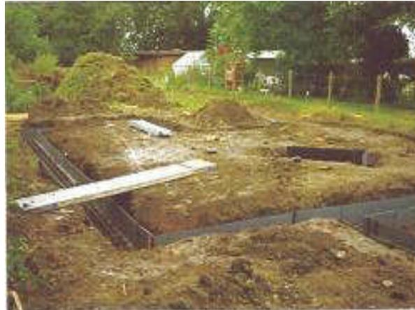
The position of the front porch and chimney base can be clearly seen above. The chimney base proved invaluable for creating the very economical "double-span" ground floor construction shown in the two pictures at the top of the next page!
