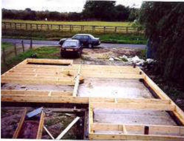
As mentioned; the foundation walls were client-built upto DPC. Then he cut and fitted the timber anchor-plate ready for the floor joists. The detailed work around the chimney base is quite impressive for a novice self-builder's first project!
