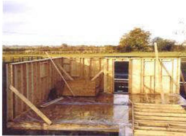
Upon our recommendation; the ground floor window openings will be left covered by the plywood sheathing; until ready to insert the windows; as a security measure. Note the next wall-panel framed and ready to receive the plywood sheathing ~ and the 'temporary braces' holding the exposed ends of the two walls!
