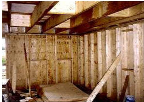
Ground floor wall-panels completed; 1st floor joists framed up, but still retaining some braces on the longer wall lengths until the floor sheathing is laid!
