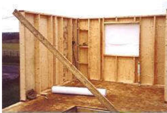
Ground floor breather-membranes can be attached quite easily without scaffolding - so that will be done after the timber-frame and roof carcassing is completed and the house has been made weather-tight!
