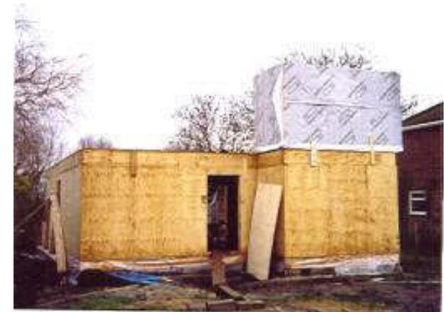
Apart from attaching the breather-membrane; the 1st floor wall-panels repeat the ground floor erection process! The window openings aren't sheathed under the breather-membrane as making a secure "enclosure" isn't necessary at 1<sup>st</sup> floor level.
