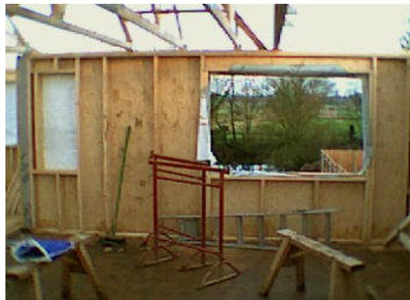
The lack of "lintels" also reduces the weight of the wall-panels; especially at the top; thereby making it easier to erect them if working single-handed as the ProFrame<sup>®</sup> system is designed to allow for!
