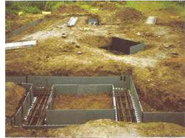
The piling is completed and the "plastic" shuttering is already in place around the steel reinforcement "cages" ready for the concrete ground beams to be cast!
