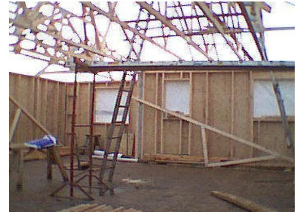
These two internal views also show two of only three openings (out of twenty-three in all) that actually required "lintels" using the ProFrame<sup>®</sup> system - saving time and money!
