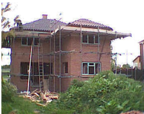
Brick cladding completed and roof tiling well advanced. Windows are fitted although the large "French" doors at rear of living room cannot be fitted until the scaffolding is removed!
