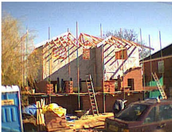
A fine sunny day sees the same front view (left) as seen on the previous page (middle-left) while the rear view is seen right. The breather-membrane is finished; window openings are visible; and the brickwork is proceeding. Windows should have been in but the "brickies" arrived first! The roof is nearly ready for fascia-boards to be fitted.
