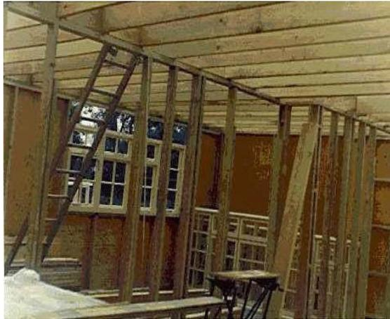
The first floor wall-panels also went together quickly; although neither the 'scenario' nor gable panel construction shown right has ever been repeated; e.g. roof-trusses are always erected before the gable-ends for both safety and peace of mind; whilst the panel construction has also radically changed since this first project!
