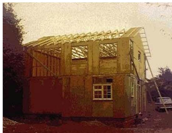
The facing brickwork to the house gable ends, entrance porch and garage (seen below right) was done by sub-contractors who supplied, erected and removed their own scaffolding over a five day period whilst they were doing the brickwork!
