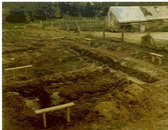
Being started during the hot summer of '76; every single brick had to be 'dunked' in a bucket of water before being laid on the mortar bed; especially as the front & back walls were just single-skin (half-brick thick) brickwork. It not only saved brickwork but also meant the foundation wall only needed a narrow 'slim-line' concrete footing beneath!
