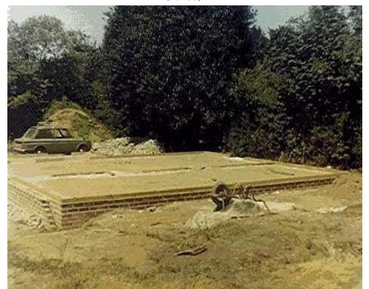
Having used the 'cutting schedule' to pre-cut all the timber and plywood sheathing for the entire house (off-site); nailing panels together and erecting them was a quick, simple process!
