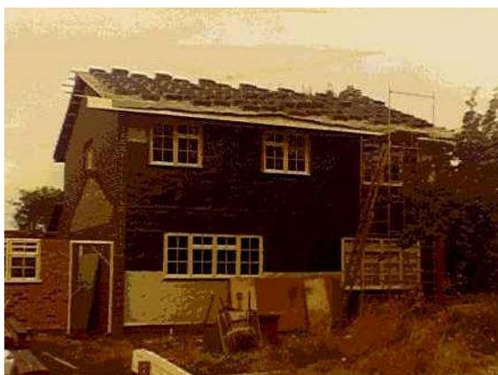
Fascia and barge-boards were all fixed working from inside the timber-frame; as was the felting and battening ~ apart from the last little 'bit'. A 'DIY' tower scaffold was used to make 'loading out' quicker and safer. (The tiles were literally carried up a ladder and stacked on the platform, four at a time, making four piles of twelve before being taken, four at a time, to load out the roof ~ five tons of them in all ~ over a single weekend.) The actual tiling was very easy by comparison.
